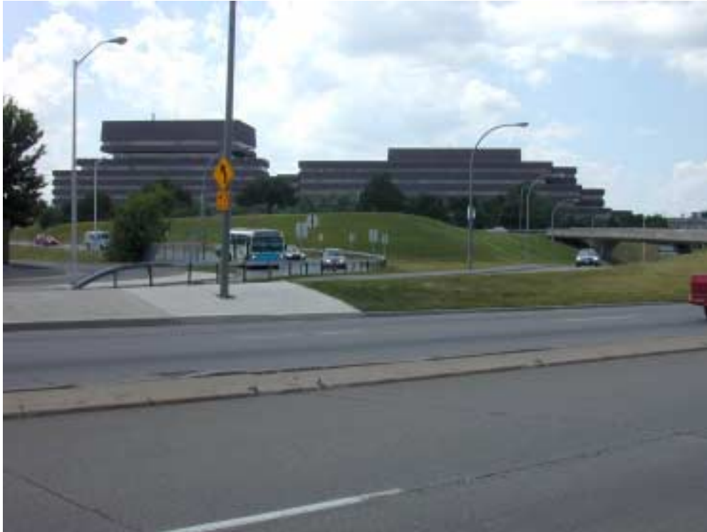
PHOTOGRAPH 19: RECEPTORS 22 AND 23, TRIANGULAR FIELD DEFINED BY KING EDWARD RAMPS AND EXTERNAL AFFAIRS BUILDING, RESPECTIVELY, LOOKING WESTWARD
