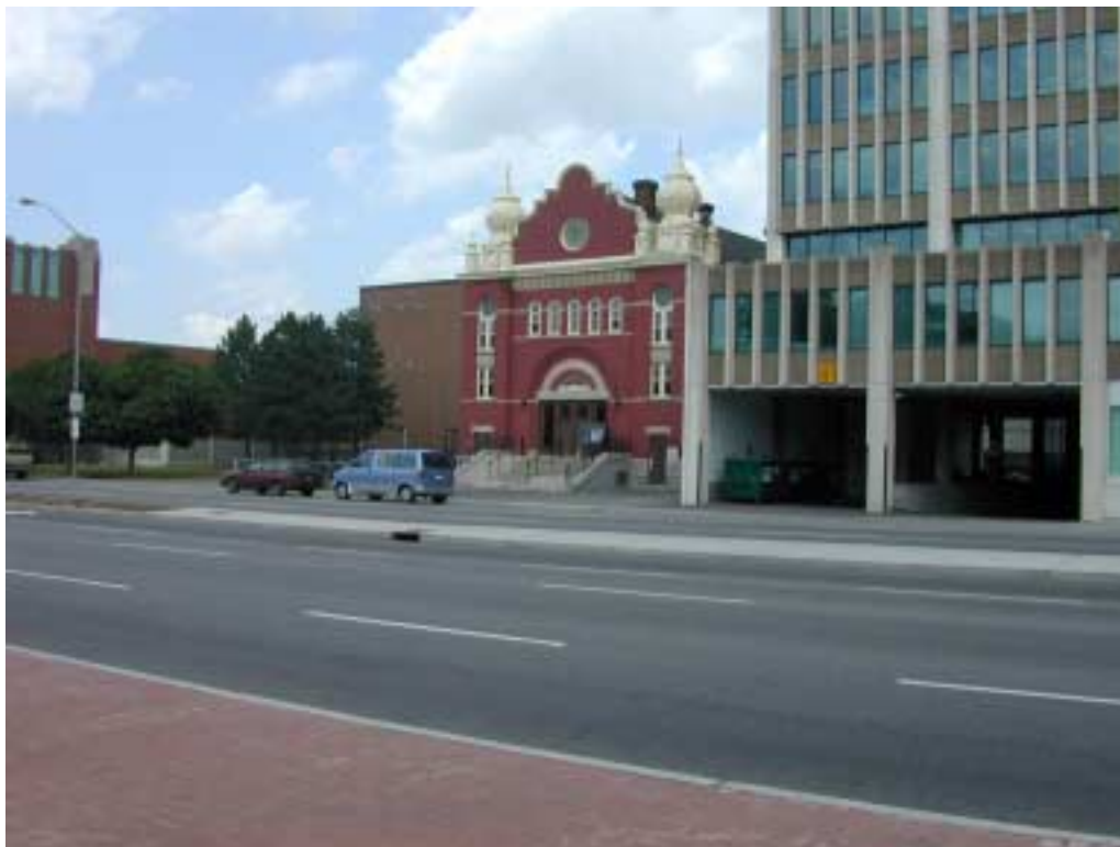
PHOTOGRAPH 8: RECEPTOR 10, 375 KING EDWARD AVE, LOOKING NORTHWARD
